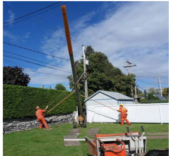
Planting a new pole
